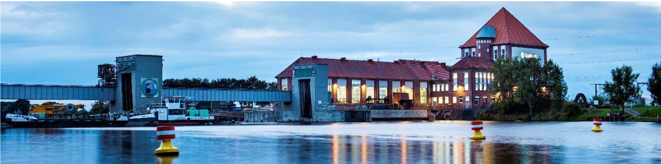
Dörverden hydropower plant, Germany
